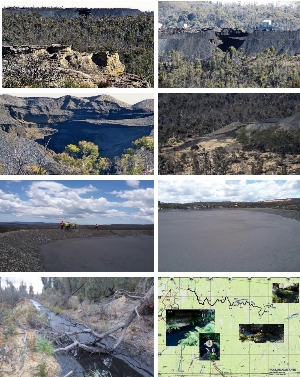
Photos: Clarence Colliery Reject Emplacement Area ("REA") 3 collapse on 2 July 2015
