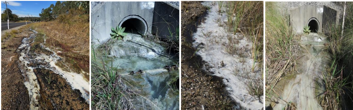
Photos 12-14: Salt discharge along Castlereagh Hwy near Mt Piper Power Station – 9 April 2016
