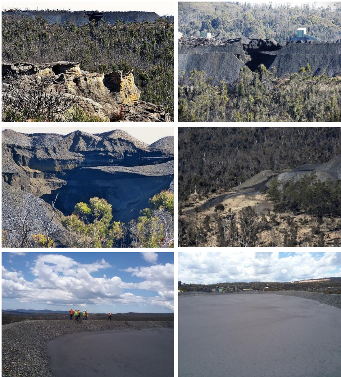
Photo 4-11: Clarence Colliery Reject Emplacement Area ("REA") 3 – collapsed on 2 July 2015
