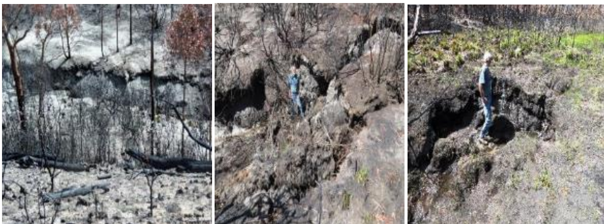
Photos 40, 41, 42: Site 12 – Erosion, scouring, slumping after undermining by Panel 707 and State Mine Fire – 24 November 2013
