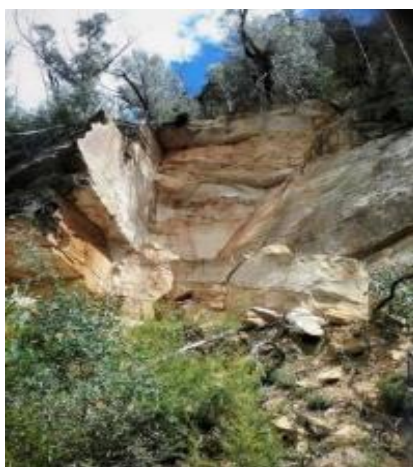
Photo 29: Cliff collapse - Panel 912
