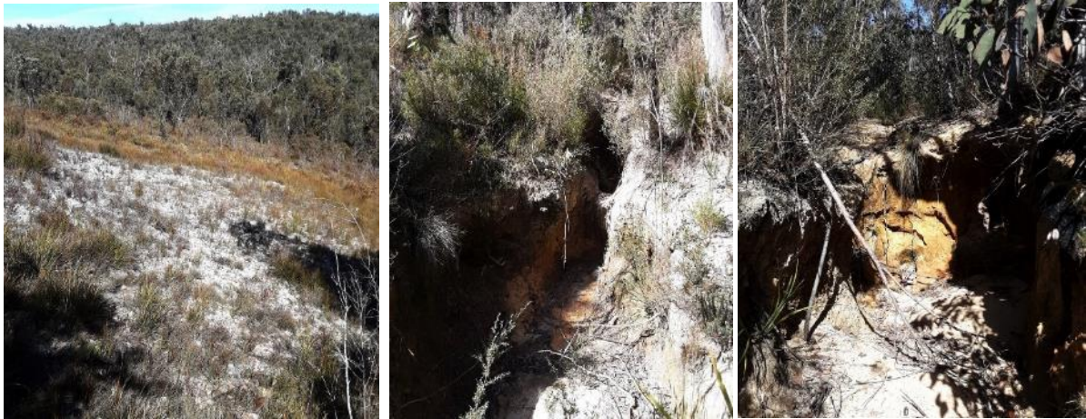
Photo 52-55: Site 14 - Dead hanging Swamps, dried up creek, possible sinkholes, severe erosion
