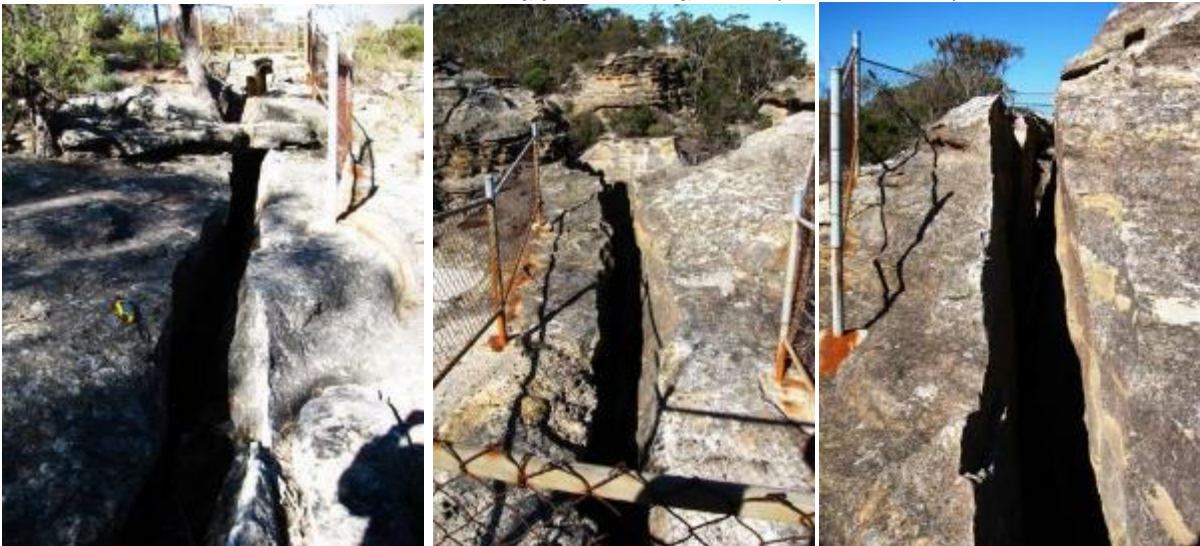
Photos 13, 14, 15 - Mine subsidence cracks – Hassans Walls Reserve – May 2009
