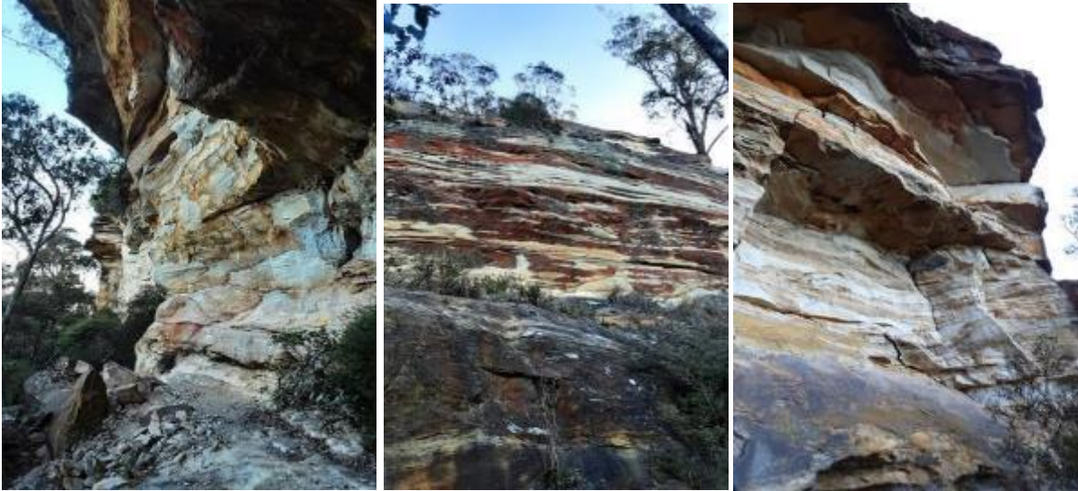
Photo 10, 11, 12: Hassans Walls cliff falls - Undercliff Track – photos taken 1 July 2023
