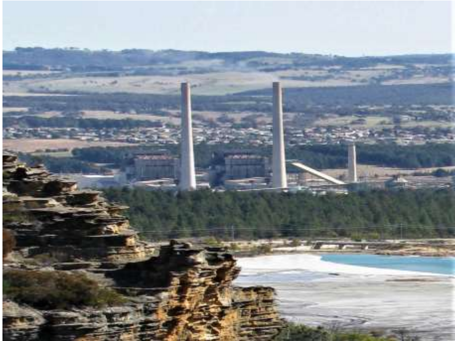
Photo: Wallerawang Power Station when operating showing the 176 metres high Unit 7 & 8 stacks, and smaller 80 metres high stack of the old Wallerawang Plant A on the right. Note Wallerawang township in the background, and smoke emissions blowing at almost right angles from stacks at 1016m elevation.
