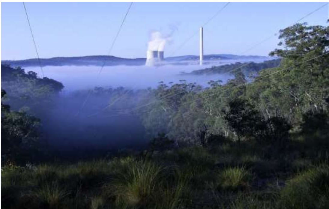
Photo: Temperature Inversion at Mt Piper Power Station. This was in January. The ERP Plant chimney at 70 metres tall is not high enough to penetrate through Temperature Inversions.
