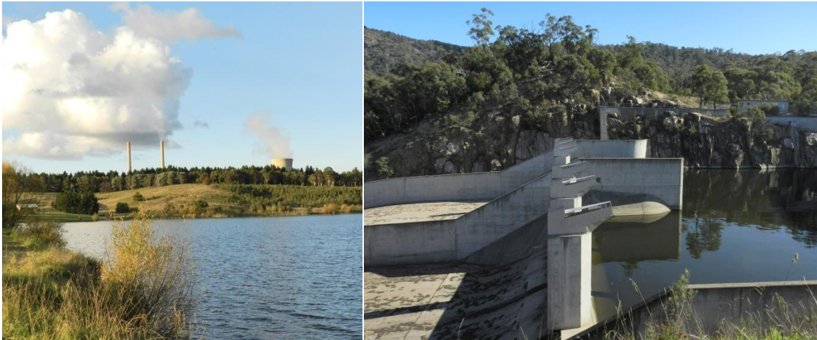
Fig. 5. The Coxs river impoundments at Lake Wallace beside the Wallerawang power station (left) and at Lake Lyell (right). These human engineered lakes are significant modifications to the Upper Coxs River freshwater system.
